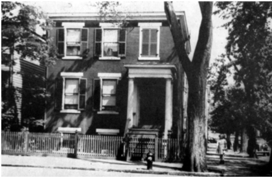
Fig. 45. 801 North Twenty-fourth Street Built 1855
