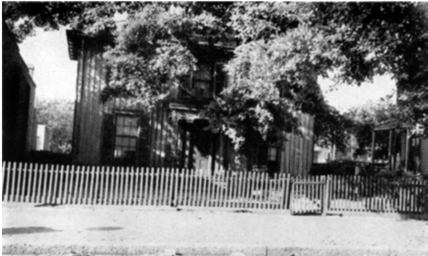
Fig. 190. 1905 West Cary Street Built 1862, Demolished 1950
