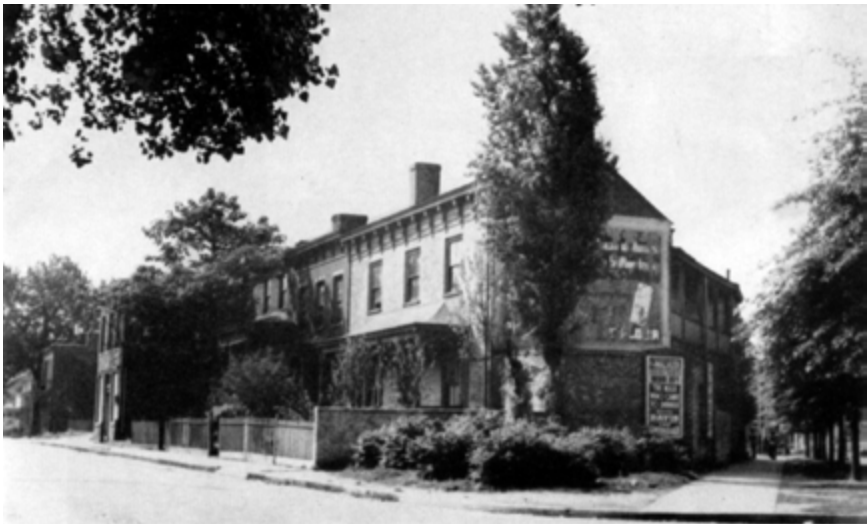
Fig. 227. Intersection of Jackson Street and Chamberlayne Avenue
