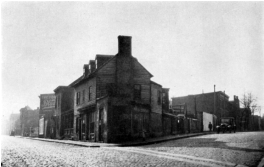
Fig. 271. Beine House 530 Brook Avenue Built 1836, Demolished 1931
