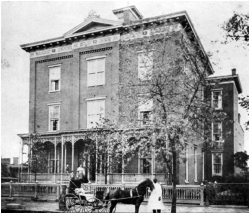
Fig. 172. Crenshaw House 21 West Main Street Built 1862, Demolished probably 1909
