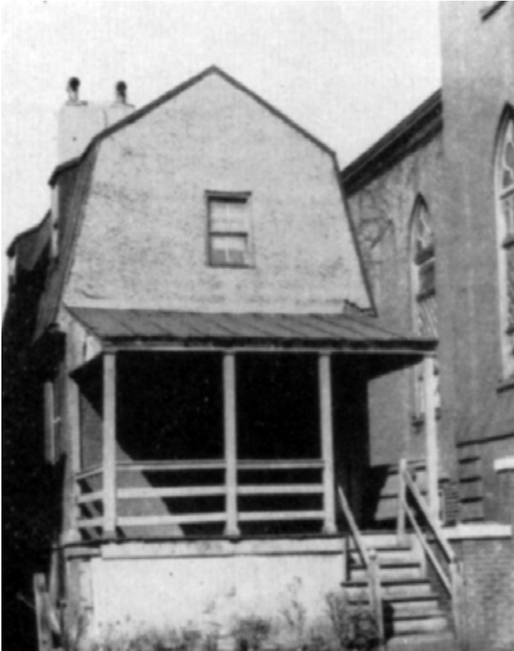
Fig. 257. 612 North Fifth Street Built 1800
