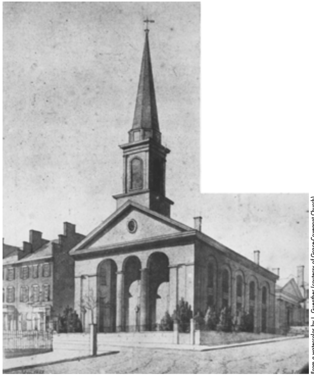
Fig. 140. United Presbyterian Church Northwest corner of Eight and Franklin Streets Built 1821, Demolished 1865
