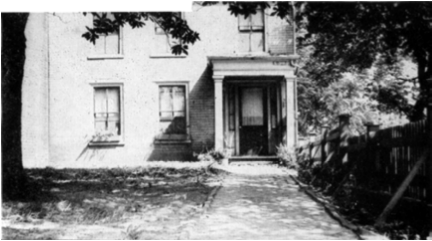
Fig. 164. 221 South Third Street Built 1848
