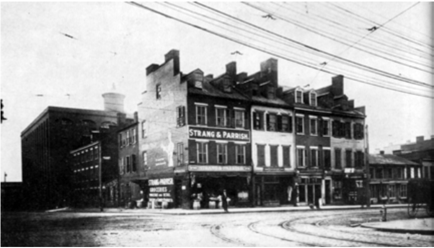
Fig. 71. 1725-31 East Main Street 1725-29 built 1841, 1731 built 1845 All except corner house demolished 1917
