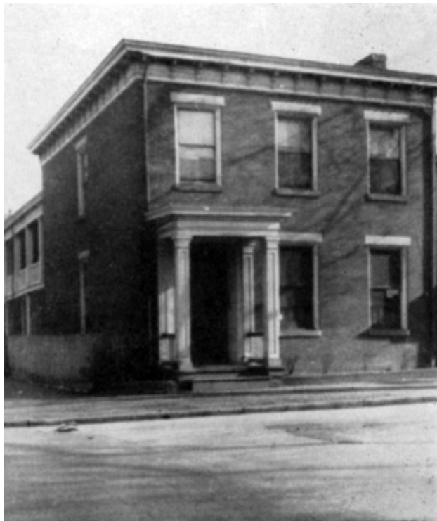
Fig. 30. Silas Johnson House 323 North Twenty-fourth Street Built 1861 or '62
