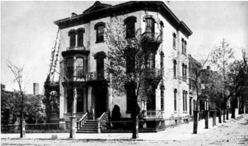
Fig. 152. Hawes House 422 East Franklin Street Built 1874, Demolished 1923
