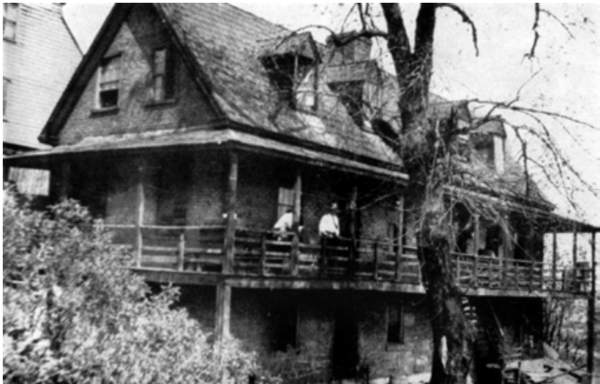
Fig. 231. Stone House on Abigail Street Date uncertain. Demolished about 1930
