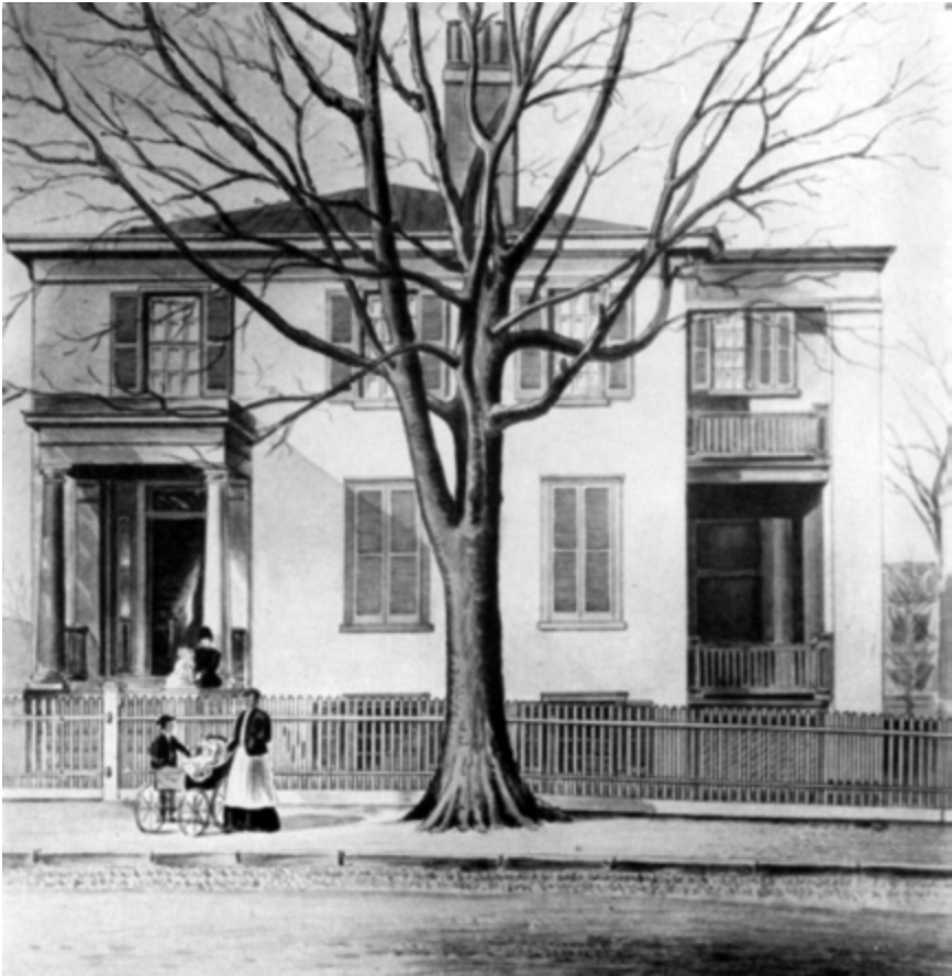
Fig. 244. Fontaine House 606 North Sixth Street Built probably in 1810, Demolished 1889
