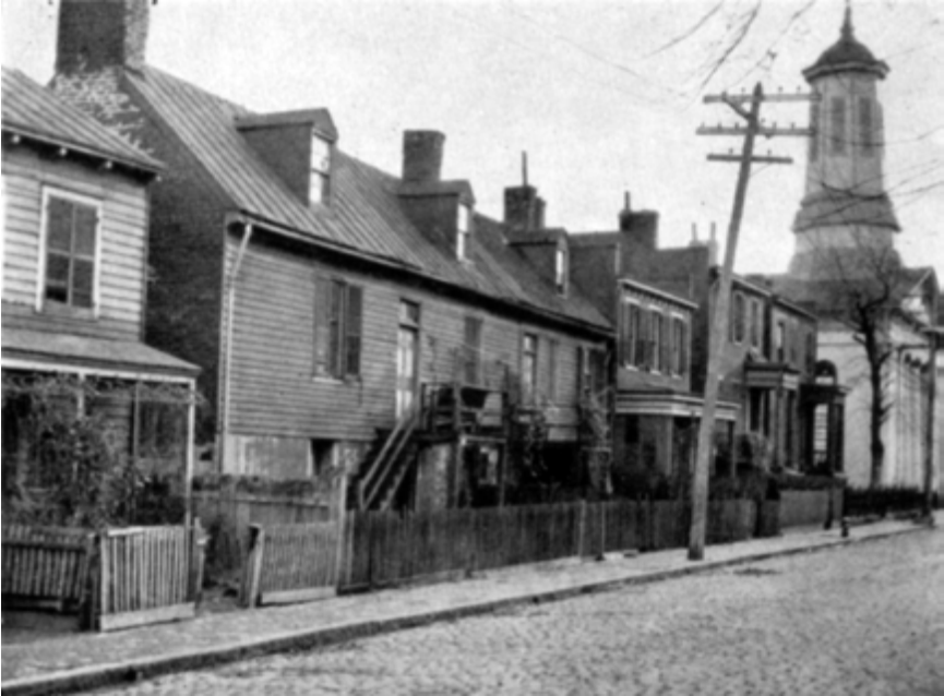
Fig. 91. 311-13 College Street Built about 1827
