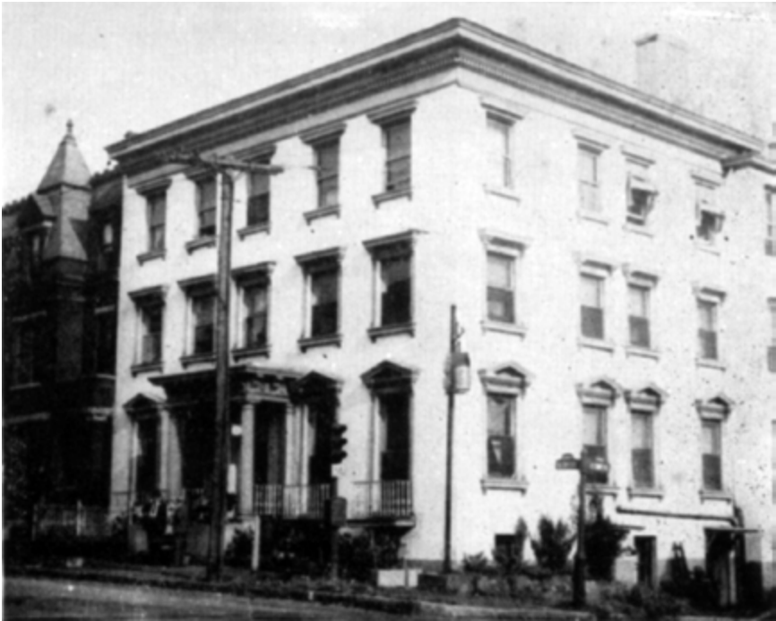
Fig. 162. 17 South Third Street Built 1809, Enlarged 1894
