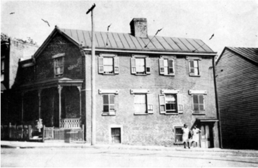
Fig. 46. Mettert House 1801 Venable Street Built between 1805 and 1811
