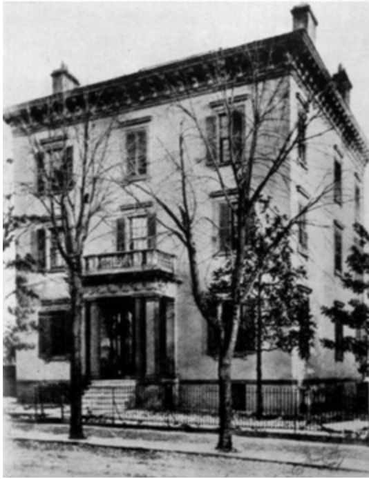
Fig. 93. Eustace-Grant House 407 North Twelfth Street Built before 1826, Demolished 1893
