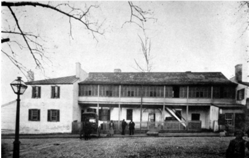
Fig. 270. Goddin's Tavern 821 Brook Avenue Built probably about 1791, Demolished 1912
