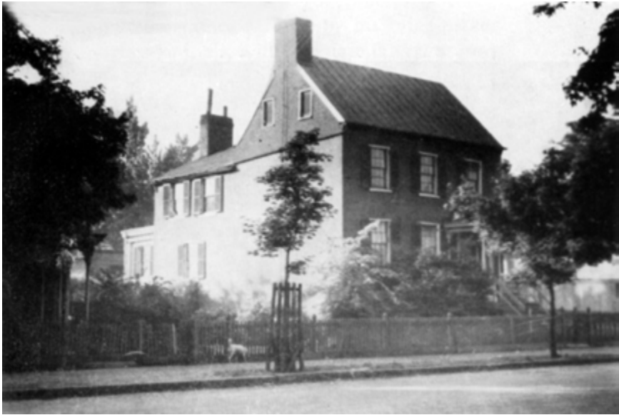
Fig. 21. Parkinson House 501 North Twenty-seventh Street Built 1818
