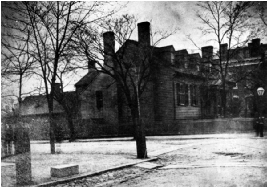
Fig. 125. Ellis House 117 East Franklin Street Built 1798, Demolished 1883
