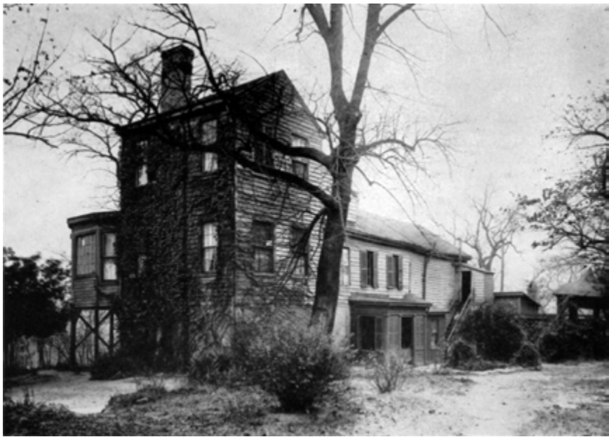
Fig. 35. Strecker-Hassel House 1904 Pleasants Street Built 1844, Demolished 1925
