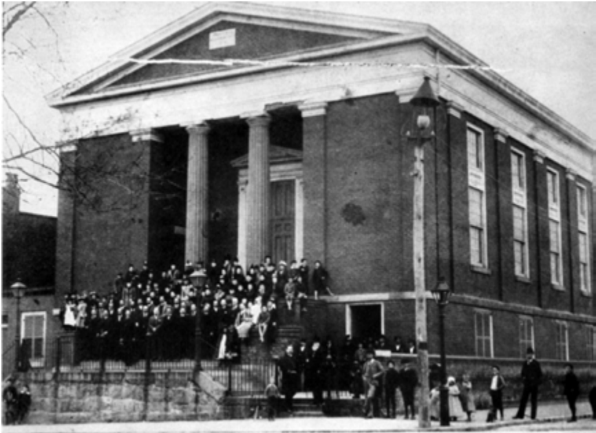
Fig. 37. Union Station Methodist Church (second building) Southwest corner Twenty-fourth and N Streets Built 1854, Demolished 1893
