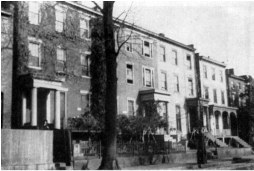
Fig. 219. 802-8 East Leigh Street Built 1855-58, Demolished 1936 and 1945
