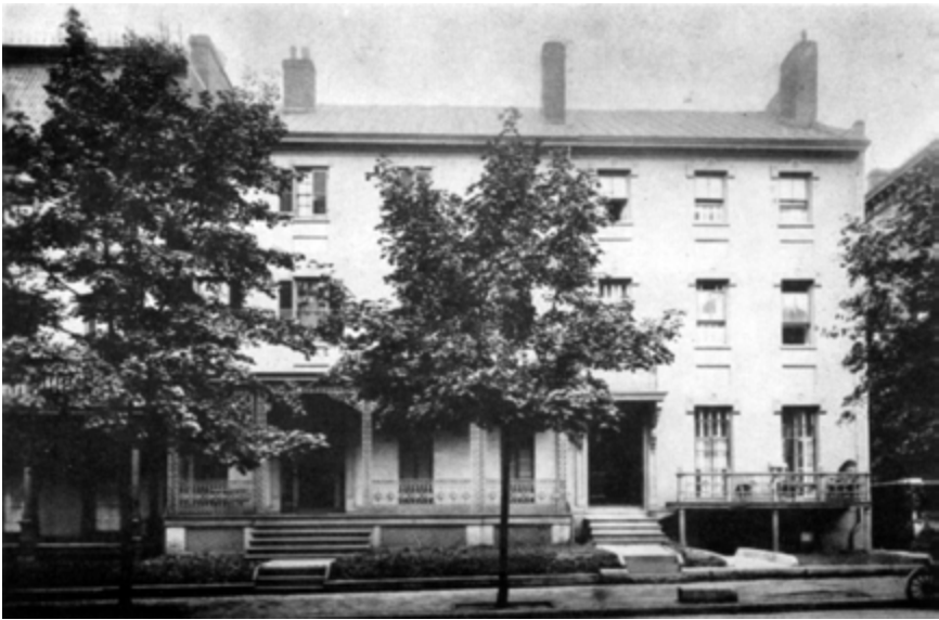
Fig. 128. 507-9 East Grace Street Built 1817, Demolished 1925
