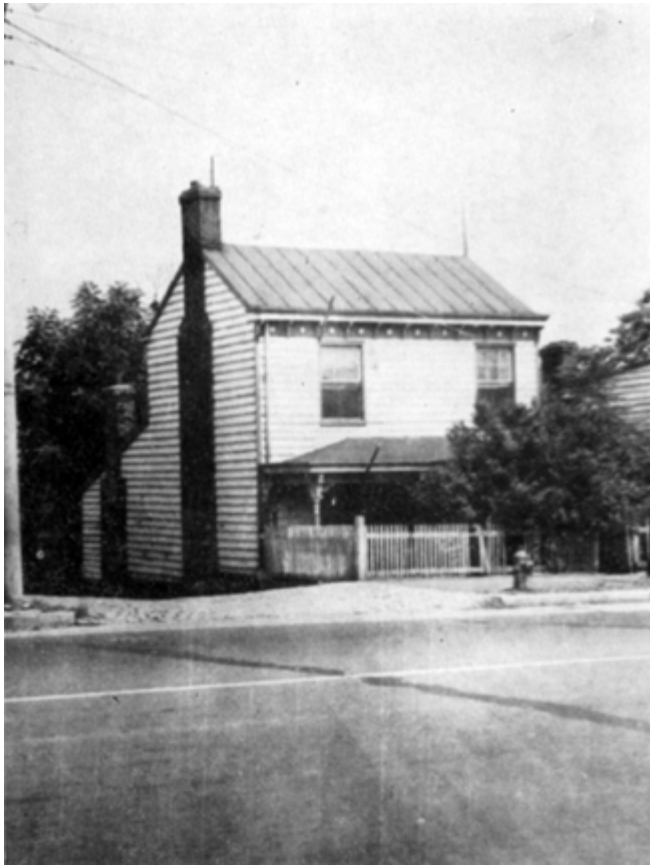
Fig. 184. 611 South Belvidere Street Built 1860
