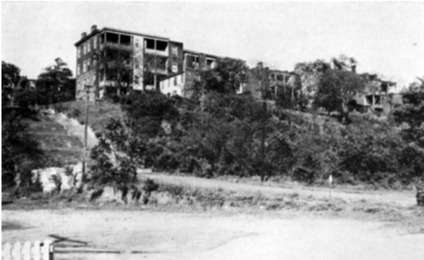
Fig. 31. Rear view of 2600 block, East Franklin Street Built in late 1850's
