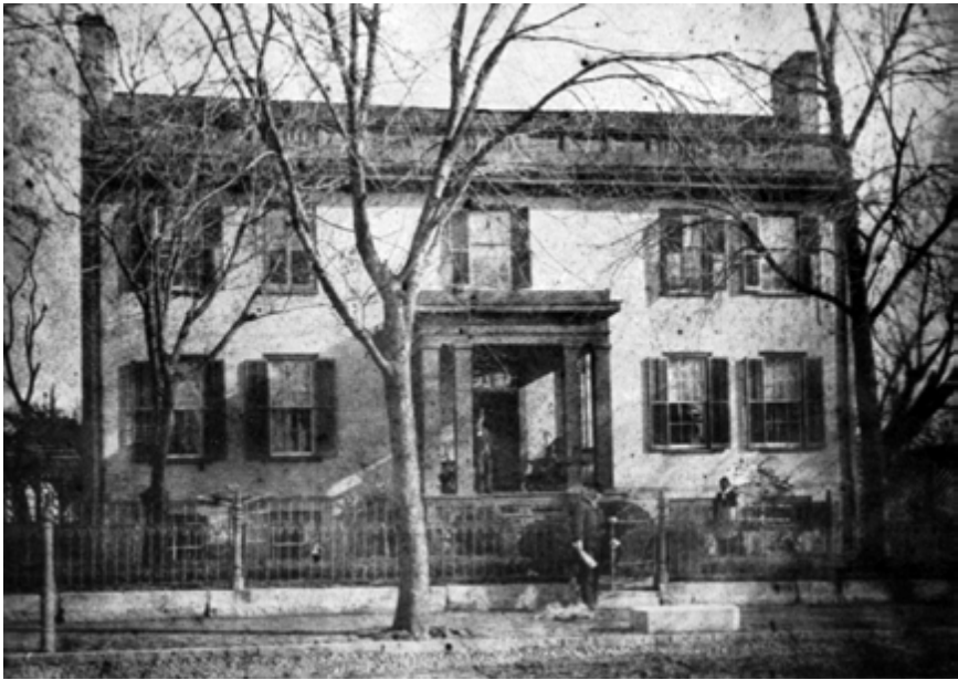
Fig. 17. 2710 East Grace Street Built 1809, Demolished 1902
