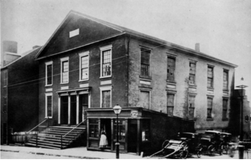
Fig. 106. Trinity Methodist Church (first building) 1417 East Franklin Street Built 1836, Demolished 1905
