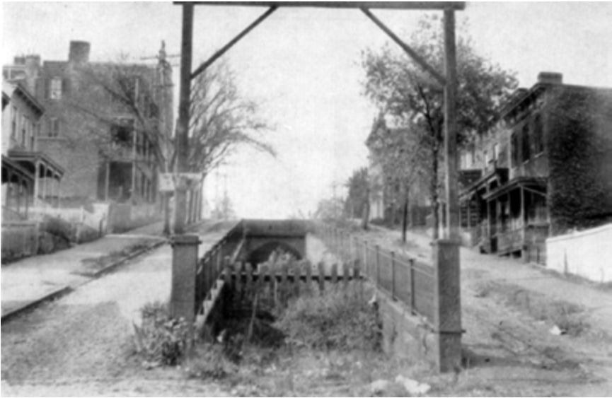
Fig. 165. Railroad Connection Tunnel Byrd Street 1867-1941
