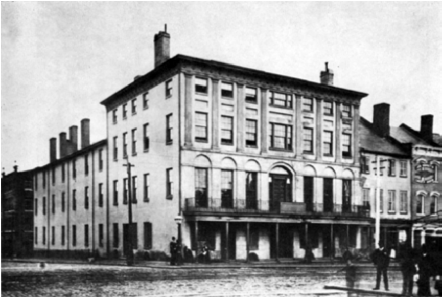
Fig. 56. Union Hotel Southwest corner Nineteenth and Main Built 1817, Demolished 1911
