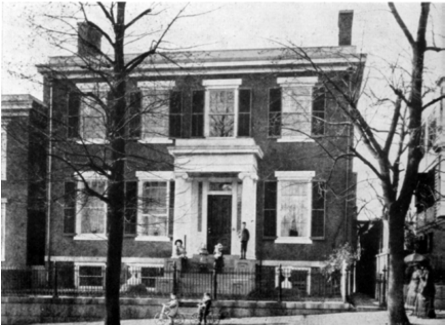
Fig. 158. Strother-Gray House 8 South Fifth Street Built 1847, Demolished 1924
