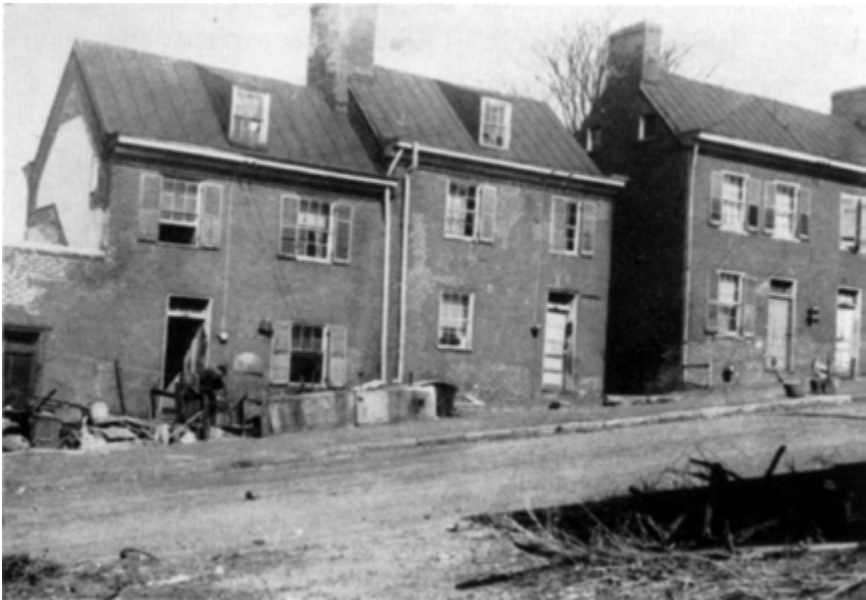
Fig. 177. Tyree Houses 208-14 South First Street Built 1841 and 1861
