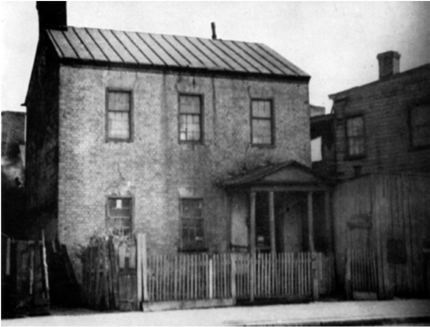
Fig. 266. Elizabeth Galt House 1001 St. James Street Built 1815
