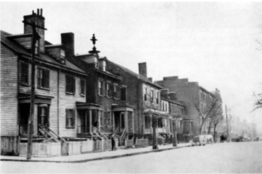
Fig. 67. Southeast corner Nineteenth and Grace Streets
