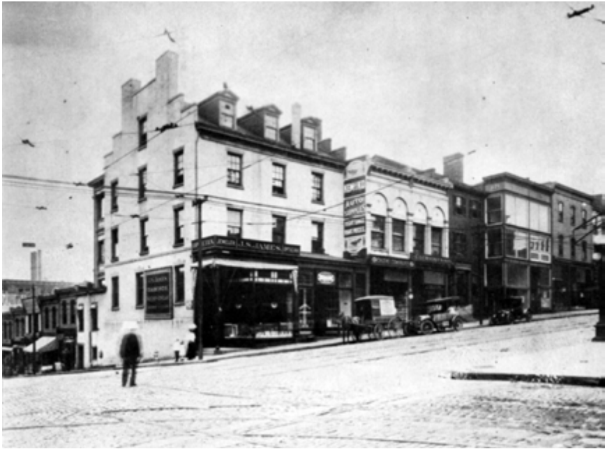
Fig. 113. Green House 631 East Main Street Built 1814, Demolished 1922
