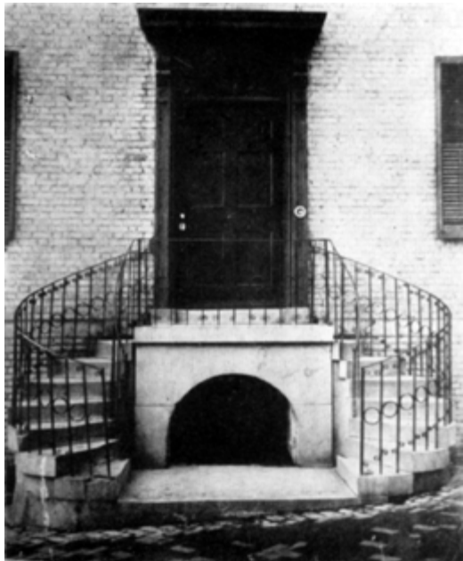
Fig. 114. Doorway of Green House
